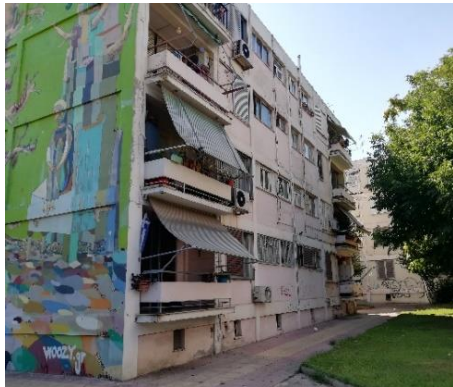
Figure 6: External view of the examined building
