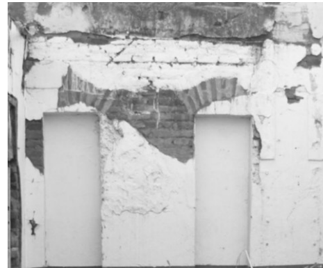
Figures 12: Current state of the former Melipilla prison.
