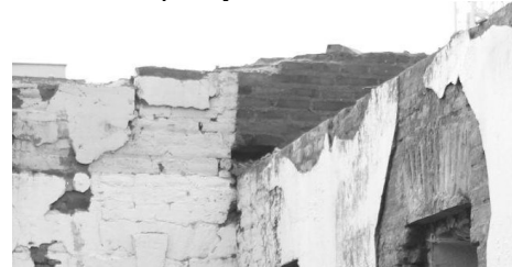
Figures 11: Current state of the former Melipilla prison.
