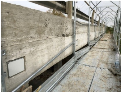
Figure 10: The positioning of the sensor on the bridge. Note the integration of the sensor into the jacketing layer.
