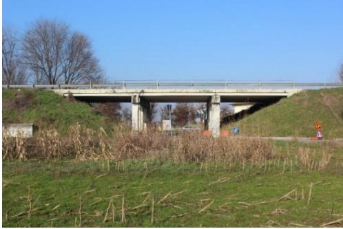
Figure 2: The status of the bridge before the renovation. Rear.
