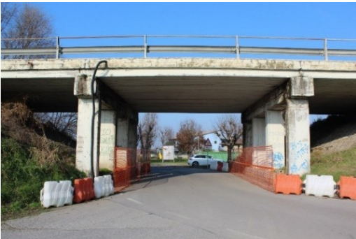
Figure 3: The status of the bridge before the intervention. Front.
