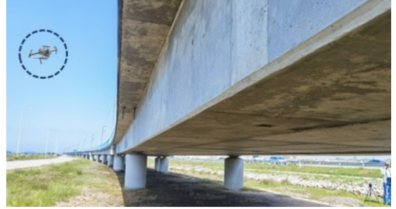
Figure 6: UAV in operation
