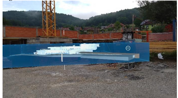
Figure 7: Display of the entire 3D BIM model of the building with its surroundings on the construction site
