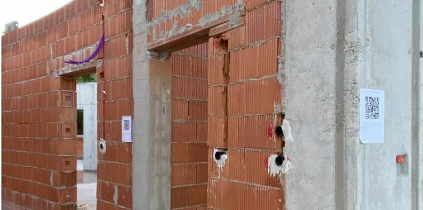
Figure 4: Attached QR codes on the building
