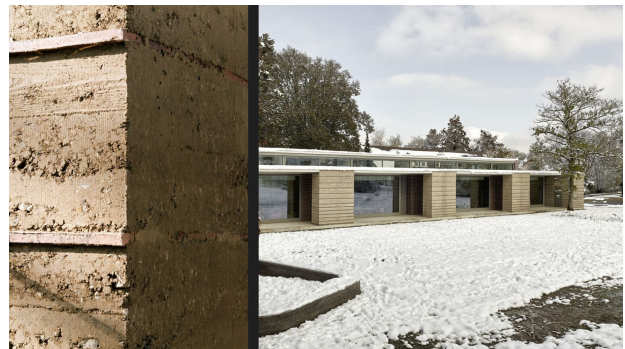
Figure 4: Umbau Schulpavillon Allenmoos II: school with rammed earth walls in Zurich © Boltshauser Architekten
