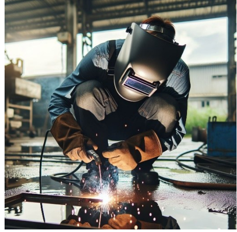
Figure 6: Case 1: Welding on Wet Floor (Generated by Microsoft Copilot)
