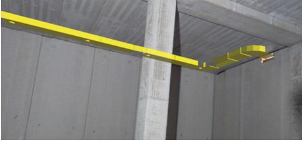
Figure 4. Module 2 weekly scheduling in AR of the installation of air exchange pipes in sector 3
