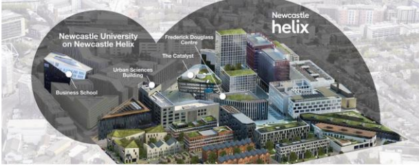
Figure 2 - Newcastle HELIX innovation district (UK)
