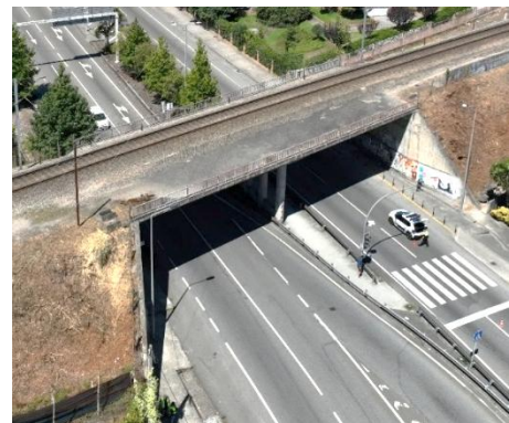
Figure 7: Aerial view of the bridge located in Porto (Portugal) used for experimental validation.
