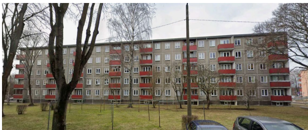
Figure 1: Example of a typical 5-storey 111-121 series building
